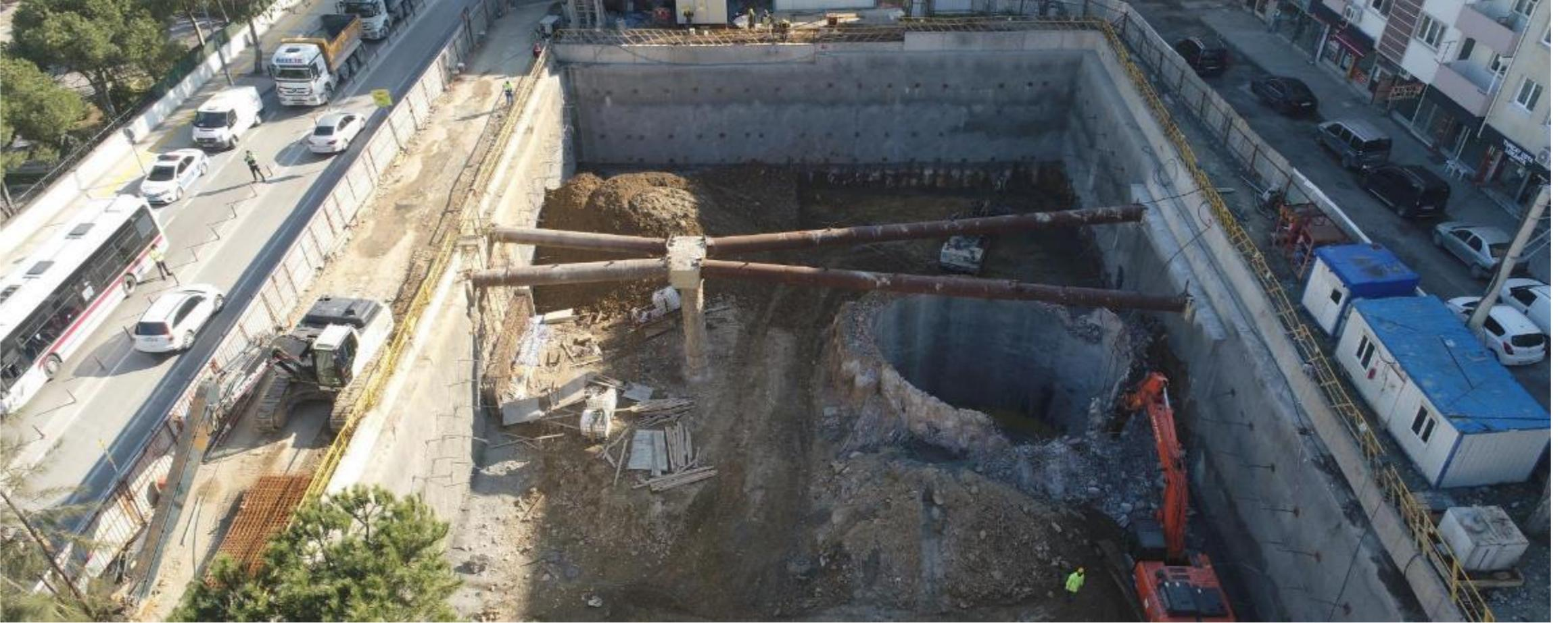
Narlıdere Station concourse structure pile fabrication has been completed. The station excavation works continue.
