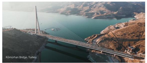
Kömürhan Connection Tunnel and Bridge is 4th in its class having 380 mt single span single pylon cable-stayed bridge of the World.
