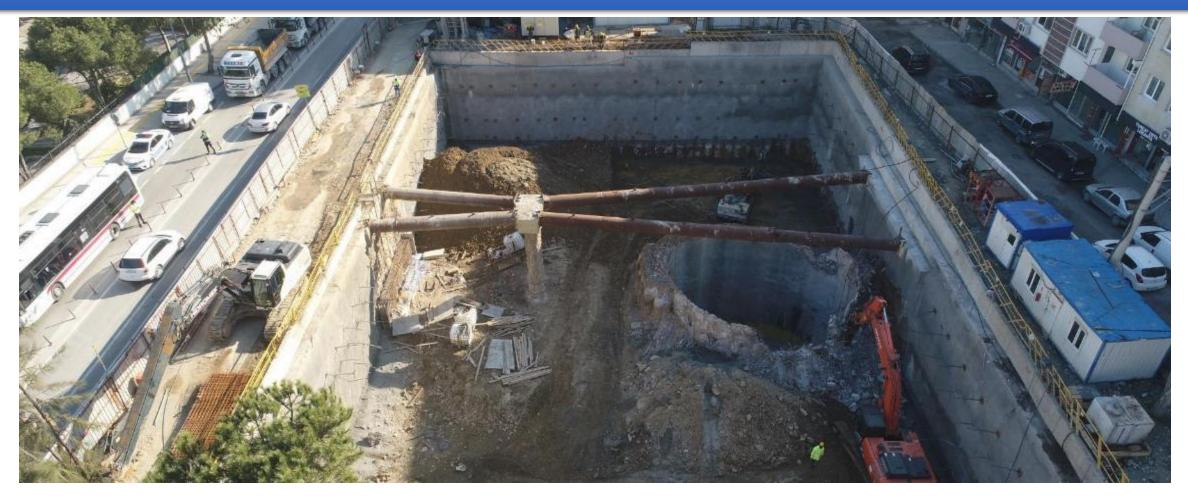
Narlıdere Station concourse structure pile fabrication has been completed. The station excavation works continue.
