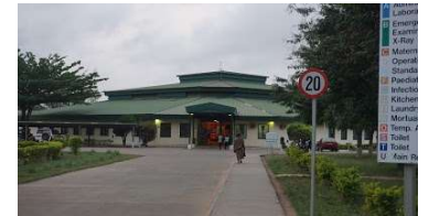
District Hospital Sogakope
